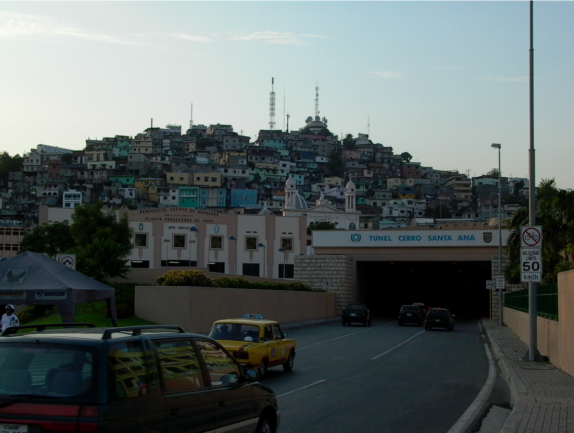
Túnel cerro Santa Ana, Guayaquil (Ecuador)
